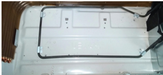
Figure 6: Outdoor Unit Drain Pan Heater.
