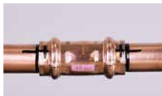
3. Mark the completed joint
