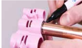
7A. Mark insertion depth on tube using depth gauge
