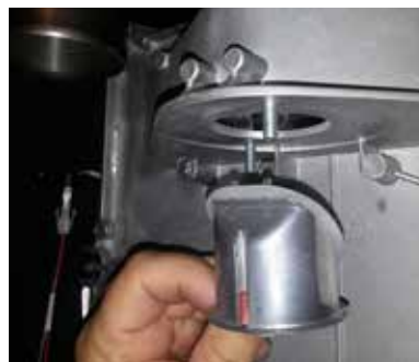
Figure 35B: Blower (EBM) and Gas Valve Assembly (HC/DC 15-95 only)
