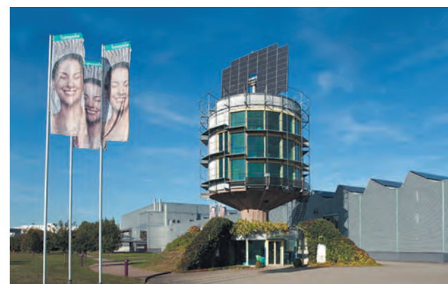
Hansgrohe’s facility in Offenburg, Germany receives a significant amount of its power from solar panels.
