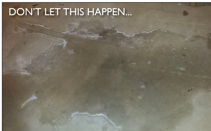
Without Polydrain, moisture can wick through the concrete and condensation puddles will form on the new floor.
