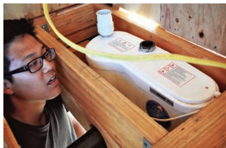
Testing of Sanigrind Pro with connecting drain pipes.
