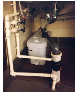
Sanivite installed underneath the counter sink
