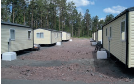
Temporary camp site with Sanicubic 1 systems
