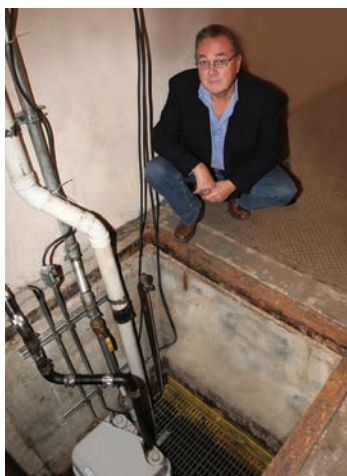
Sanicubic 2 grinder pump installed inside a pit where several bathrooms drained into the pump
