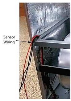
Figure 23: Reinstall Coil Assembly.
