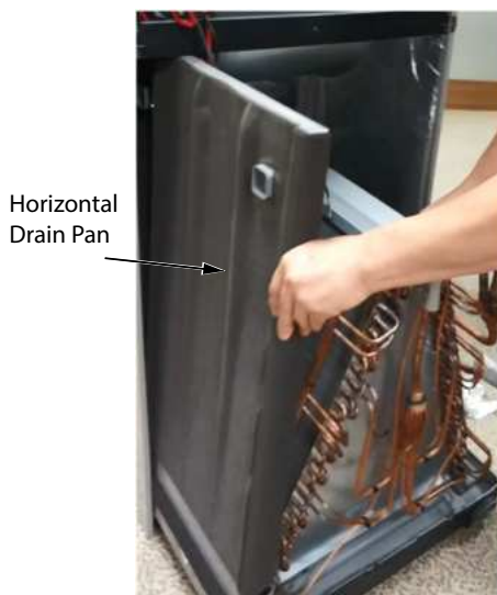
Figure 18: Evaporator Coil/ Drain Pan Assembly.
