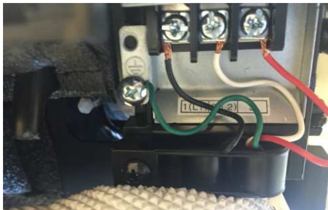
Figure 73: Typical Indoor Unit Terminal Block with Grounding Cable (Example Only).
