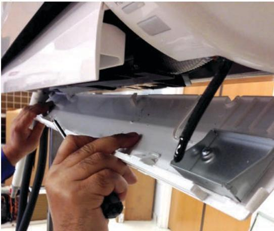
Figure 57: Indoor Unit Knockout (Communication Wires)
