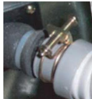
Clamp the Flexible Drain Hose Connection
