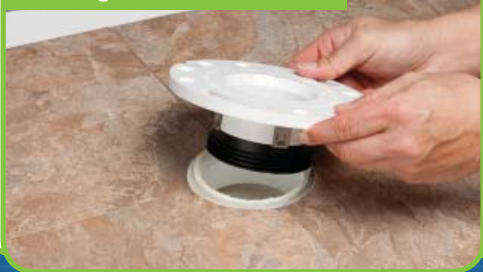
Repair Flange Fits Inside Existing Hub
