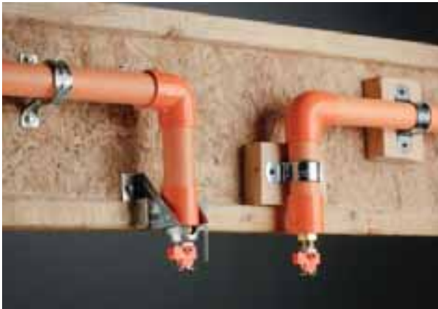
Time-saving SOSR installation depicted beside traditional labor intensive wood block assemblies.
