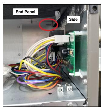
Figure 11. Electrical Connections (Upflow Configuration)
