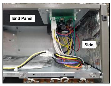
Figure 12. Control Panel Relocated to End Panel (Horizontal-Right Configuration)
