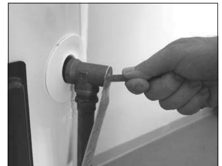
Figure 46 - T&P Relief Valve
