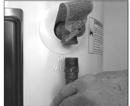
Figure 13 - Removing the T&P Relief Valve discharge pipe.
