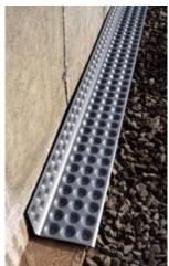
6. The area should then be backfilled as soon as possible, taking care not to over-impact.
