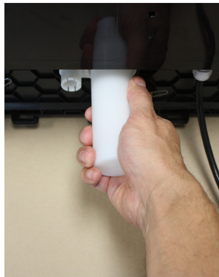
Figure 17: Condensate trap installation
