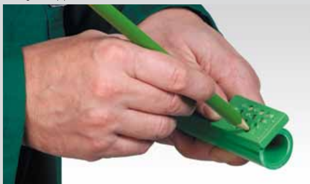
Marking of the welding depth
