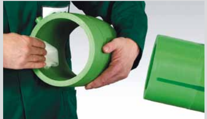
Clean the electrofusion socket's inner surface with a lint-free cloth or paper. Remove moisture that may occur immediately before the welding process again.
