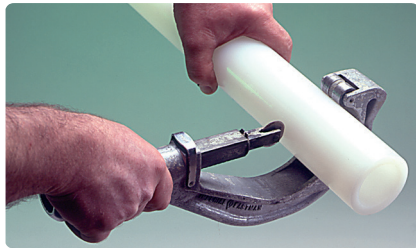
Figure 4-24: Cut the Pipe
