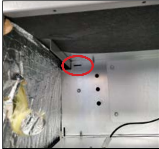
Figure 4. Notch for Control Panel Relocation
