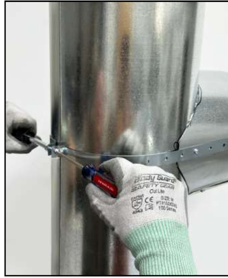
EXAMPLE OF STRAPPING COLLAR TO FLUE PIPE
