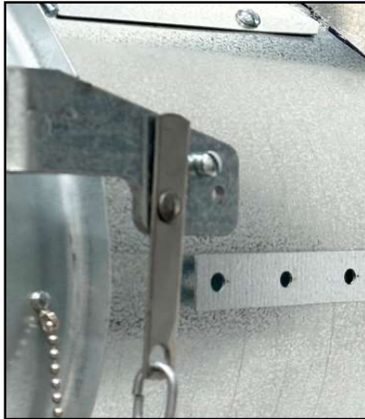
SCREW POSITION VERTICAL INSTALLATION
