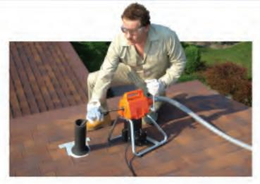
for small drain work, the drum stops turning when you lift the handle to the neutral position.
